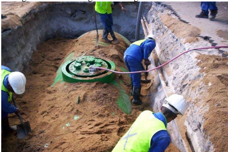
Backfilling around an underground storage tank with selected material:
