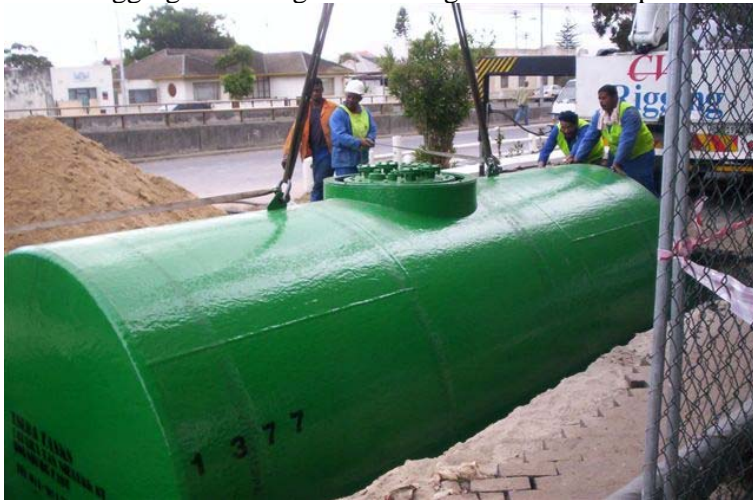
Backfilling around an underground storage tank with selected material:
