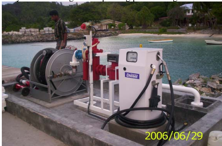
Jetty fuel receiving and dispensing point during installation:
