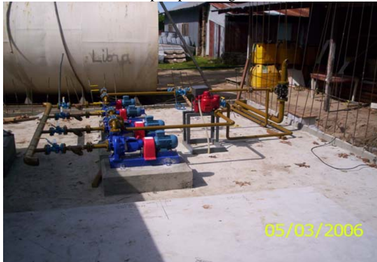
Distribution pumps during installation:
